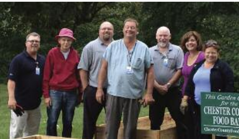
GREEN TEAM MEMBERS FINISH RAISED GARDEN BED CONSTRUCTION OUTSIDE OF THE HOSPITAL
